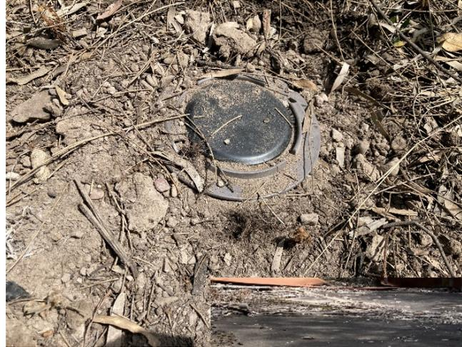
White Ant treatment stations are installed at ground level at regular spacings around the building and routinely monitored.
